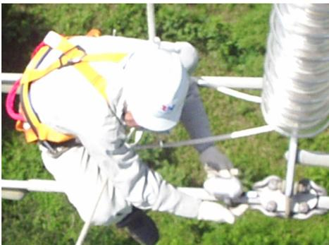
Figure 2. Equipment installation on the energized conductor
